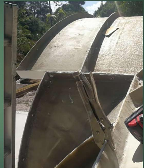
TO ACHIEVE THE RIGHT ALIGNMENT AND POSITIONING BETWEEN PANELS YOU NEED THREE PEOPLE WORKING. ONE PERSON CHECKS ALIGNMENT FROM THE INSIDE WHILE THE OTHER TWO WORK ON THE OUTSIDE CLAMPING, DRILLING AND BOLTING THE PANELS TOGETHER. THE PERSON ON THE INSIDE CHECKS FOR ALIGNMENT USING A SHORT LENGTH OF 2 X 4, RUNNING IT ACROSS THE SEAM TO VERIFY AND USING IT TO PUSH PANELS INTO ALIGNMENT.
