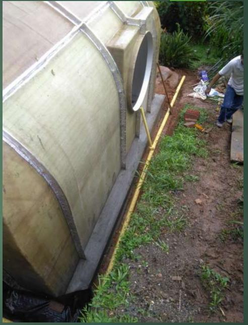
ONCE ALL INSTALLATIONS ARE FINISHED AND JOINTS SEALED, WE PROCEED TO THE FINAL SEALING OF THE DOME, ACCORDING TO THE METHOD CHOSEN, EITHER WITH EXPANDED POLYURETHANE INSULATION, A LIQUID MEMBRANE, OR OTHERS (SEE NOTES) ... IN ANY CASE, THE FINAL WATERPROOFING MUST CONTINUE BEYOND THE SLAB – PANELS JOINT.
