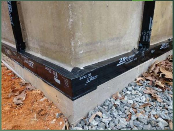
THE SECOND LAYER OF PROTECTION IS FORMED BY COVERING ALL JOINTS AND BOLTS WITH SELF ADHESIVE SEALANT TAPE, AS WELL AS FLASHING AGAINST THE SLAB.
