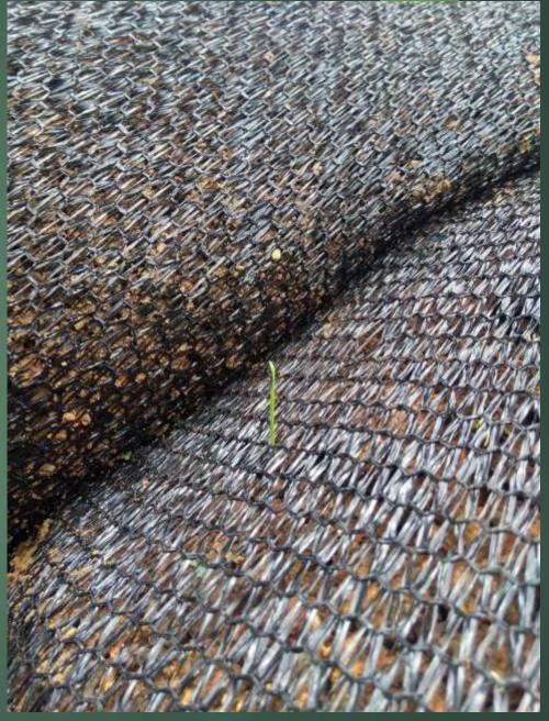
THE BAGS SHOULD BE FILLED WITH A SOIL MIXTURE THAT MUST CONTAIN 30% TOPSOIL TO FACILITATE THE GROWTH OF VEGETATION ... AT THE BASE OF THESE AND FOR SOME DISTANCE UPWARDS IT IS NECESSARY TO FILL WITH LOOSE SOIL BETWEEN THE BAGS AND THE DOME . FOR THIS YOU CAN USE THE EARTH FROM THE EXCAVATION OR OTHERS THAT ALLOW MANUAL COMPACTION WITH A HAND TAMPER.
