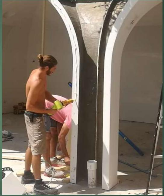
WE THEN ALIGN THE PANELS TOGETHER AND BEGIN FIXING THEM IN POSITION WITH VISE-GRIP PLIERS.
