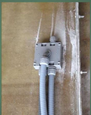
CONDUIT AND ELECTRICAL BOXES ARE COVERED ON THE OUTSIDE OF THE PANELS WITH THE DUCT COVERS THAT COME WITH THE KIT. THESE ARE GLUED TO THE MODULES WITH THE SAME ADHESIVE SEALANT USED THROUGHOUT THE ASSEMBLY.
