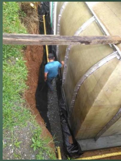
ONCE THE FILTERS ARE FINISHED AND THE SHELL IS SEALED, WE CAN BEGIN TO FILL IN WITH EARTH WHERE NECESSARY AND STRUCTURE THE BERMS OR EARTH WALLS. FOR BERMS THAT HAVE MORE THAN 45 DEGREES OF INCLINATION AND ARE ABOVE GROUND LEVEL, WE RECOMMEND THE BAG SYSTEM DESIGNED BY BIOTEKT. THESE BAGS ARE MADE OF A POLYPROPYLENE MESH WITH UV PROTECTION AND ALLOW THE GROWTH OF VEGETATION THROUGH THE WEAVE...
