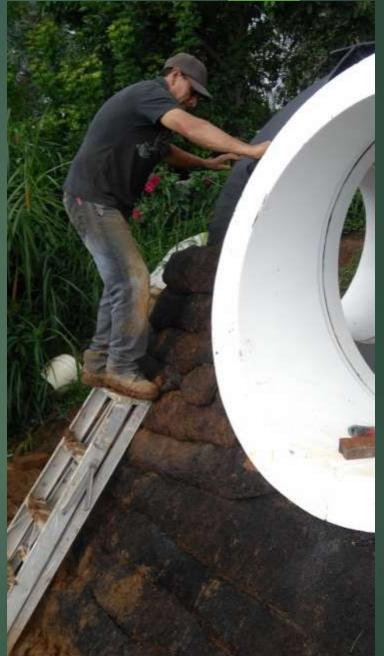
STRUCTURED BERMS SHOULD GO ALL THE WAY UP TO THE JUNCTION BETWEEN THE WALL AND ROOF PANELS. ABOVE THESE WE PLACE LOOSE SOIL. THIS MUST ALSO HAVE A MINIMUM OF 30% TOPSOIL, AND AN APPROXIMATE THICKNESS OF 30 CENTIMETERS WITHOUT COMPACTING.
