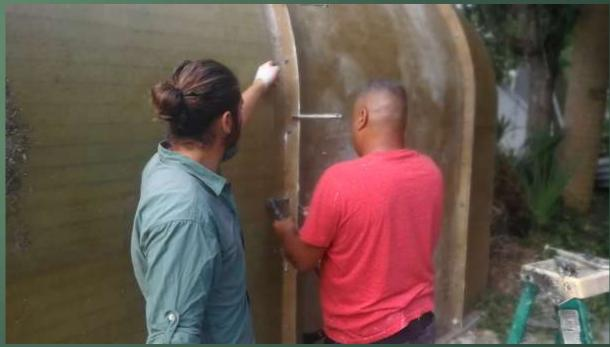
WITH SEVERAL MODULES CONNECTED TO EACH OTHER, WE CAN BEGIN FIXING THE MODULES TO THE CONCRETE... FOR THIS IT IS VERY IMPORTANT TO ALIGN AND LEVEL EACH MODULE BEFORE AND AFTER FIXING THEM TO THE FLOOR. DO NOT TIGHTEN THESE SCREWS THOROUGHLY UNTIL THE ENTIRE DOME IS ASSEMBLED. IT IS ADVISABLE TO PLACE SOME DIAGONAL BRACING TO KEEP EVERYTHING VERTICAL UNTIL THE ENTIRE SHELL IS ASSEMBLED..
