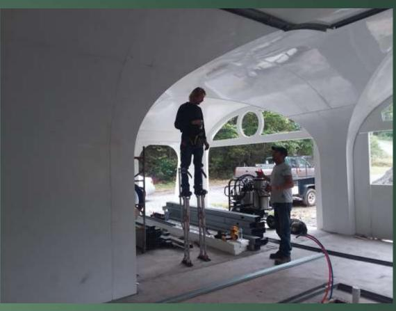
WHEN WALL AND ROOF PANELS ARE ALL IN PLACE WE CAN INSTALL WINDOW AND DOOR EXTENSIONS.
