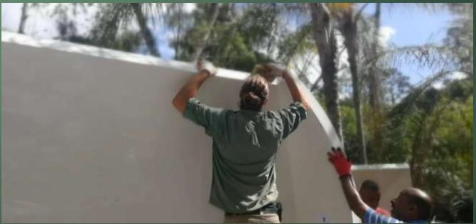
ONCE THE PANELS ARE ALIGNED AND CLAMPED TOGETHER, WE CAN START DRILLING AND FASTENING NUTS AND BOLTS... BOLTS ARE DISTRIBUTED MAXIMUM 20 CENTIMETERS ON CENTER, BEGINNING WITH THE CORNER BOLTS. ALL BOLTS MUST BE PLACED ON THE FLANGES AT MAXIMUM 3 CENTIMETERS FROM THE PANEL BODY. APPLY A BIT OF ADHESIVE IN THE HOLES IF YOU CANT SEE ANY GLUE IN THEM TO ENSURE A GOOD SEAL.
